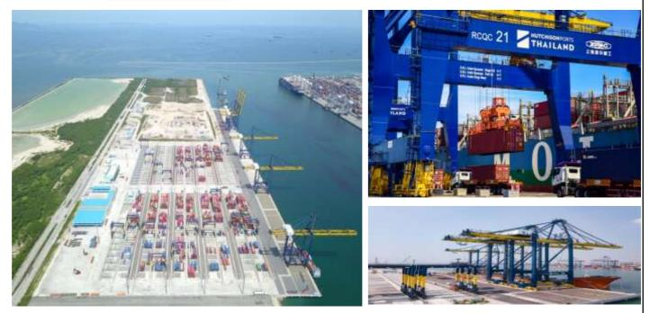
Hutchison Ports (Thailand) Ltd. has implemented the use of remote controlled Quay Cranes and Rubber Tyred Gantry Cranes (e-RTGC) in its Terminal D development in Laemchabang Thailand. Six quay cranes and twenty electrically powered e-RTGCs have successfully completed commissioning tests and are now in full operation.
